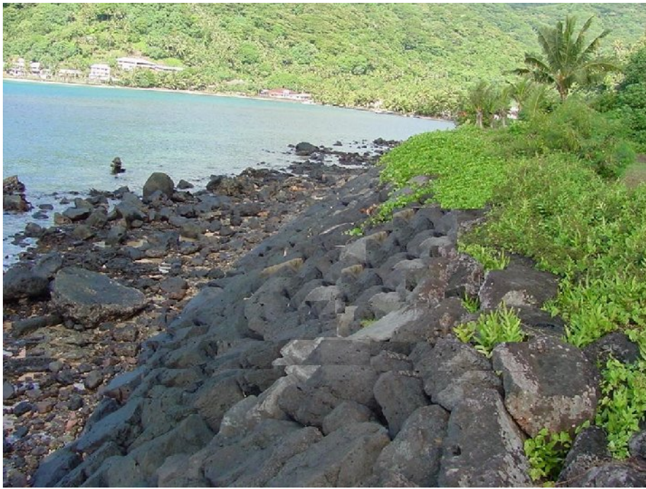
Picture 6.2.: Rock armour on the shoreline
