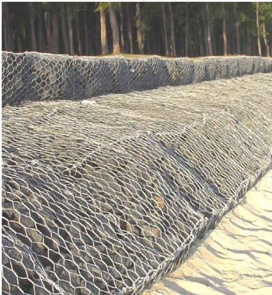
Picture 6.3.: Gabion rock revetment. Source: Baird 2003
