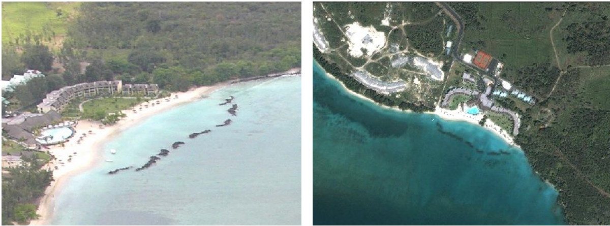
Picture 6.1. (a) & (b): Aerial and satellite image of detached breakwaters in front of The Sands Resort Source Aerial from Baird 2003, Satellite from Flash Earth
